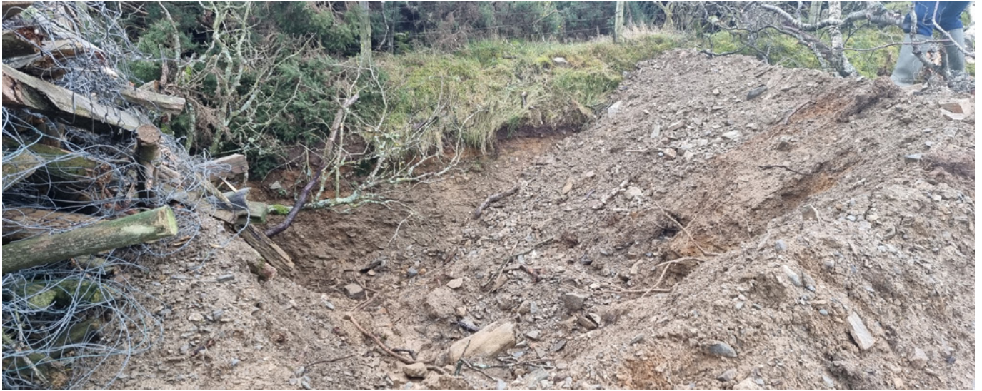
Photo: Excavation and obstruction of an unclassified road in North Wales to stop 'damaging' motorised use. The pit extends across the full width of the road and is more than 2m deep.
